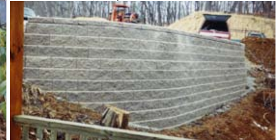
Segmented Retaining Wall
