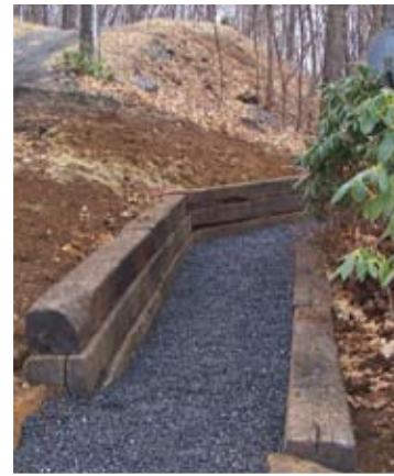
Railroad Tie Retaining Wall
