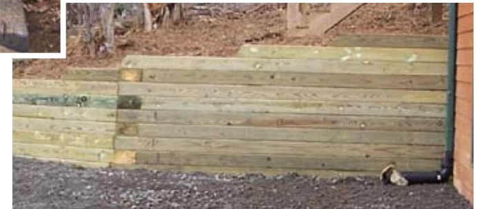
Timber Retaining Wall
